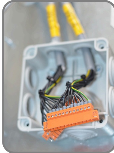
Signal connection by multipin cube in IP54 box
