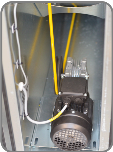
Made connection between motor and compressors
